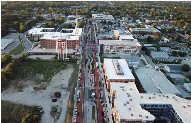
An aerial photo of some of Carmel's recent downtown development. Source: City of Carmel.
