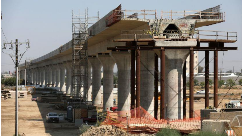
Construction of California's high-speed rail project in Fresno, Calif., in 2018.
